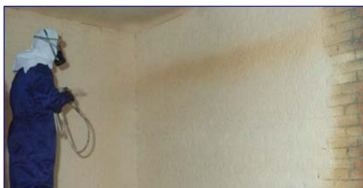
Picture 23: Spraying over a masonry wall
